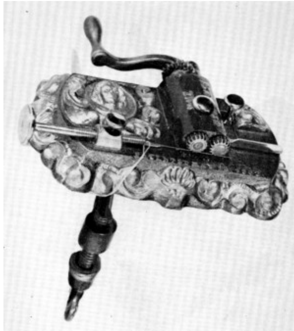
Figure 52.—THE FAIRY SEWING MACHINE sold for five dollars and was adequate for its advertised purpose, sewing or running very lightweight fabrics. The machine was marked with the Palmer patent, the date May 13, 1862, and the name “Mme. Demorest.”
