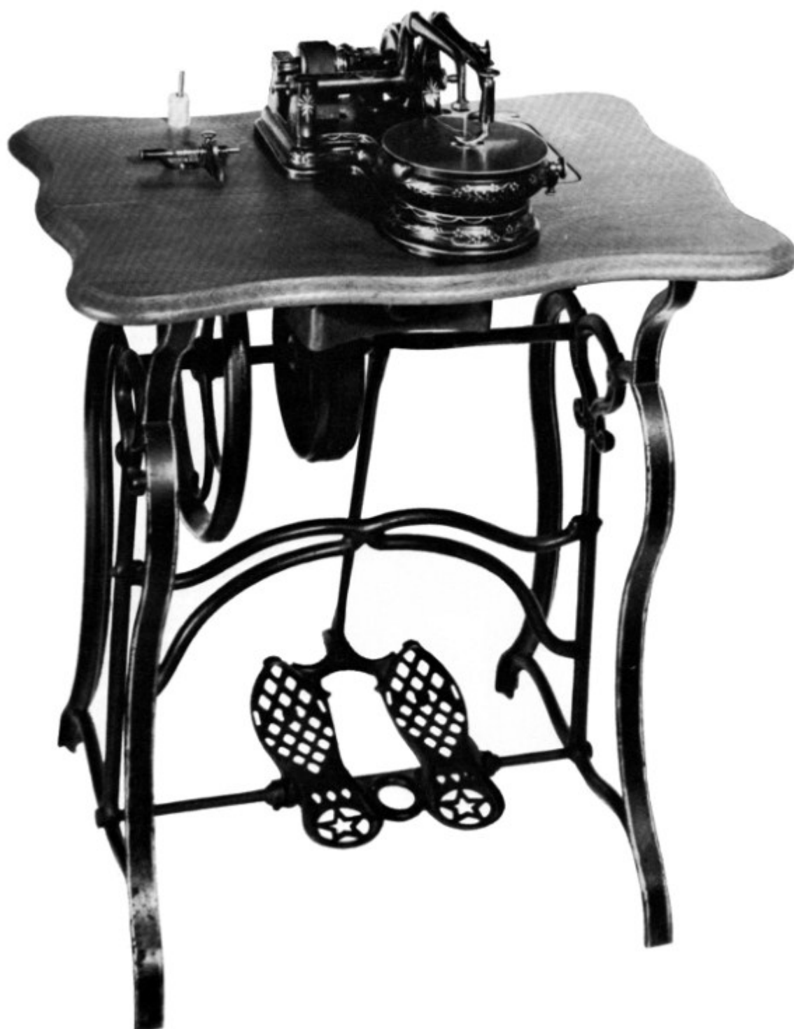
Figure 83.—FLORENCE SEWING MACHINE. The Florence machine was based on the patents of Leander W. Langdon, whose first patent was obtained in 1855. Langdon sewing machines were manufactured by the inventor for a few years. It was his patent of March 20, 1860, that was the immediate forerunner of the Florence machine, whose name
