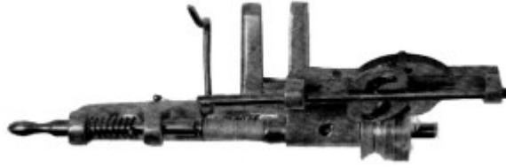
Figure 59.—SHANK'S patent bobbin winder, 1870. (Smithsonian photo P-6398.)
